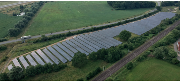
Park: Karstädt, Germany Park size: 10,0 Mwp Mounting system: FMS H6
