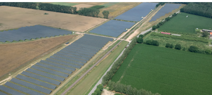
Park: Werder, Germany Park size: 8,9 Mwp Mounting system: FMS H6
